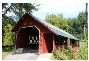
trusses, which was a popular design in covered bridges throughout New England. The timbers are fastened to one another and to the cords at the top and bottom by wooden pins. A 1920 renovation added the covered sidewalk on one side along with a slate roof to replace the original shingles.
