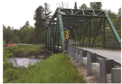
allowed construction crews to piece the bridge together entirely on site leading to quick and efficient bridge construction. Earlier truss bridges were put together at the factory, and then shipped to the construction site and installed.
