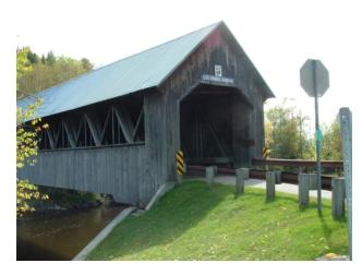
1840 by Massachusetts millwright William Howe, and with iron and wooden parts, represents the transition from wood to metal as the primary construction material for bridges. While the iron pieces helped with strength and longevity, the wooden materials kept costs down, and this lower initial cost made it an economically sound design choice.
