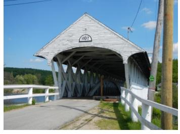
The Groveton Bridge is an example of a Paddleford truss bridge, a truss style
