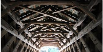
Hall Covered Bridge was replaced in 1982 with a 120-foot design of traditional materials and timber framing methods, following its 1980 collapse due to the crossing of an overweight vehicle. While Hall Bridge was entered into the National Register of Historic Places on September 20, 1973, the National Register nomination form could not be found in Vermont State files.
