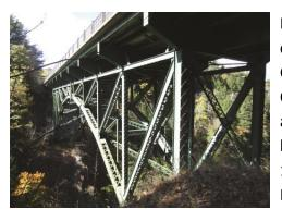
Located in a wooded area of scattered residential, commercial, and agricultural buildings in Windsor County, the Quechee Gorge Bridge (also called the Ottauquechee River Bridge) is the oldest standing steel arch bridge in Vermont. This large tri-span, spandrel-braced, deck arched bridge is 285' long, 41' wide, and sits 163' above the Ottauquechee River. The Quechee Gorge Bridge provides breathtaking views of Vermont's deepest
