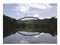
base of the arch is below the bridge deck, but the top of the deck is built above the arch, so the deck passes through the arch.
